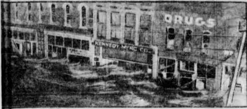
View of considerable damage was taken at individual and shows the room flood that struck Kansas, Kansas as a result of a cloudburst, which it says of its height. The picture was taken in Kansas from the rear of one of the business blocks. Water reached here than half way to second floor downtown buildings. Several were drowned before the water subsided.
