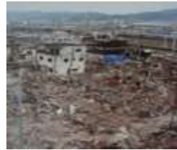
b) Hanshi-Awaji Earthquake
