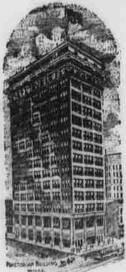
The Praetorian Building
