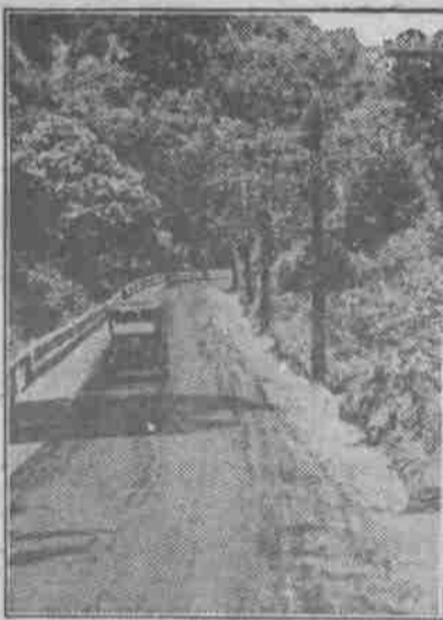
Properly Protected Road.
