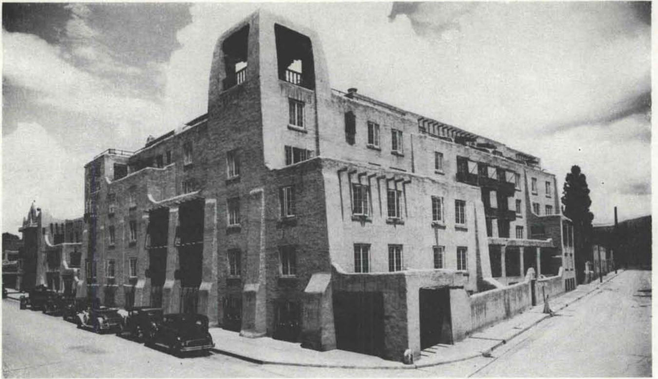
LA FONDA, Santa Fe, N. M., view from southwest.
