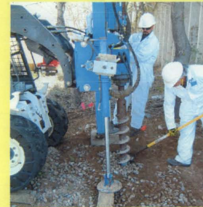
Auger drilling through the gravel aggregate to collect additional soil samples for VOC analysis at the AOC 1117 Drywell.
