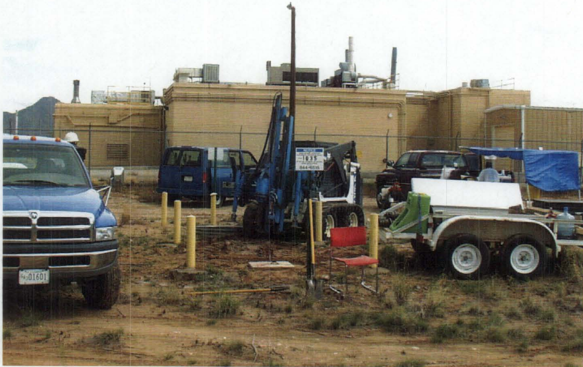
Figure 3.4-1 Collecting soil samples with the Geoprobe™ from the borehole drilled through the center of the seepage pit at DSS Site 1035, the Building 6715 Septic System. View to the southeast. September 12, 2002
