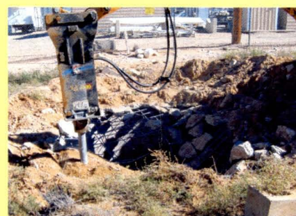
Seepage pit demolition and backfilling.
