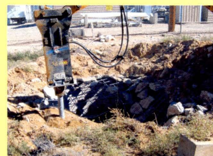
Seepage pit demolition and backfilling.
