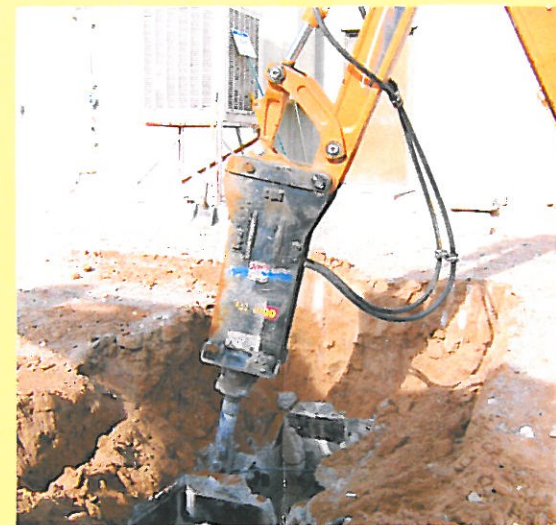
Septic system demolition and backfilling.
