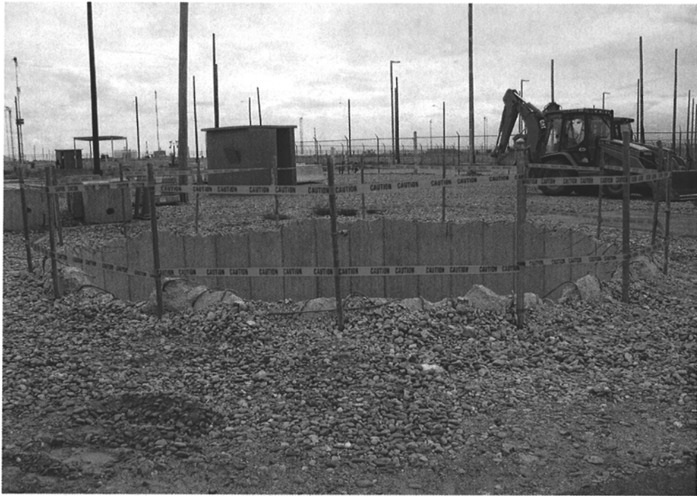
Figure 1. The above-ground portion of the Cistern wall after removal.
