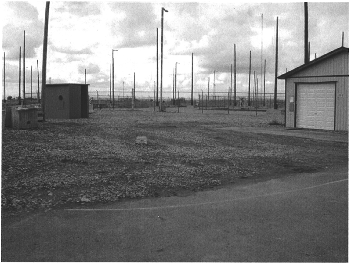
Figure 5. SWMU 196 after completion of backfilling activities.
