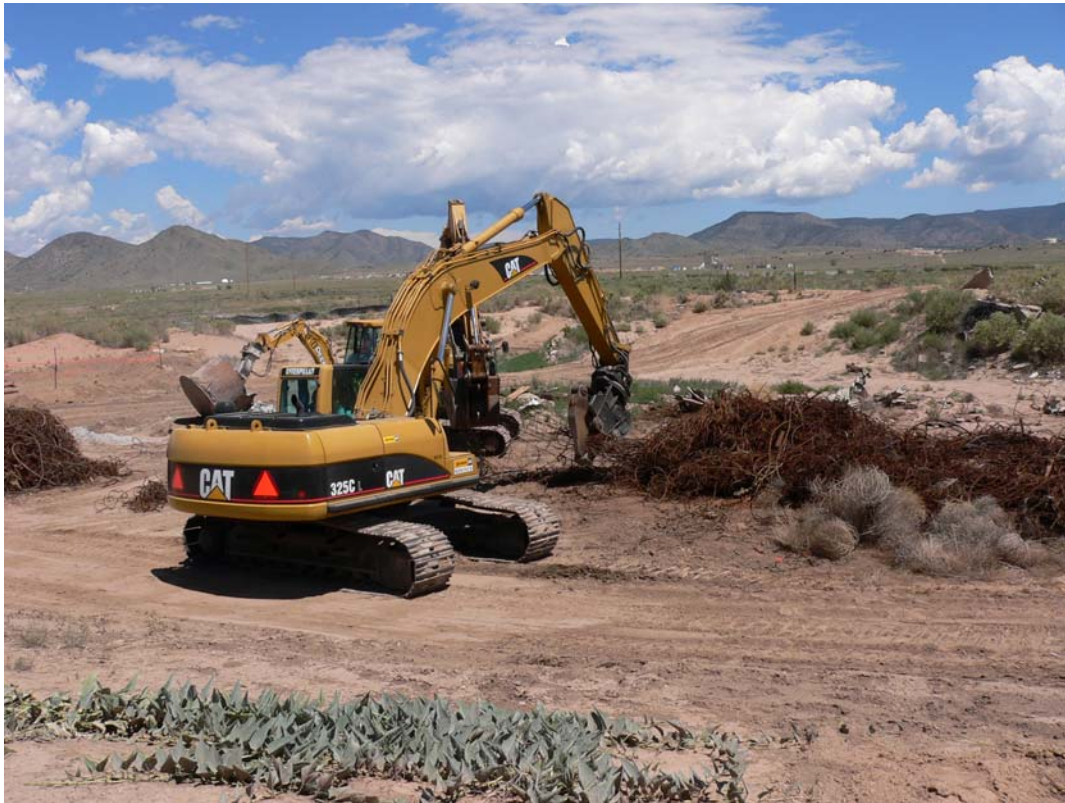
LTES Site 1 Cable Debris Removal
