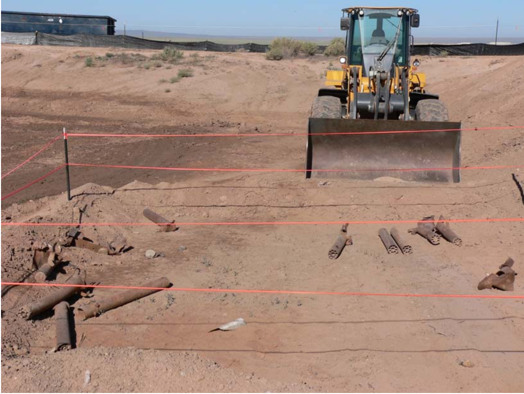
LTES Site 1 Spent 5 inch Rocket Motors
