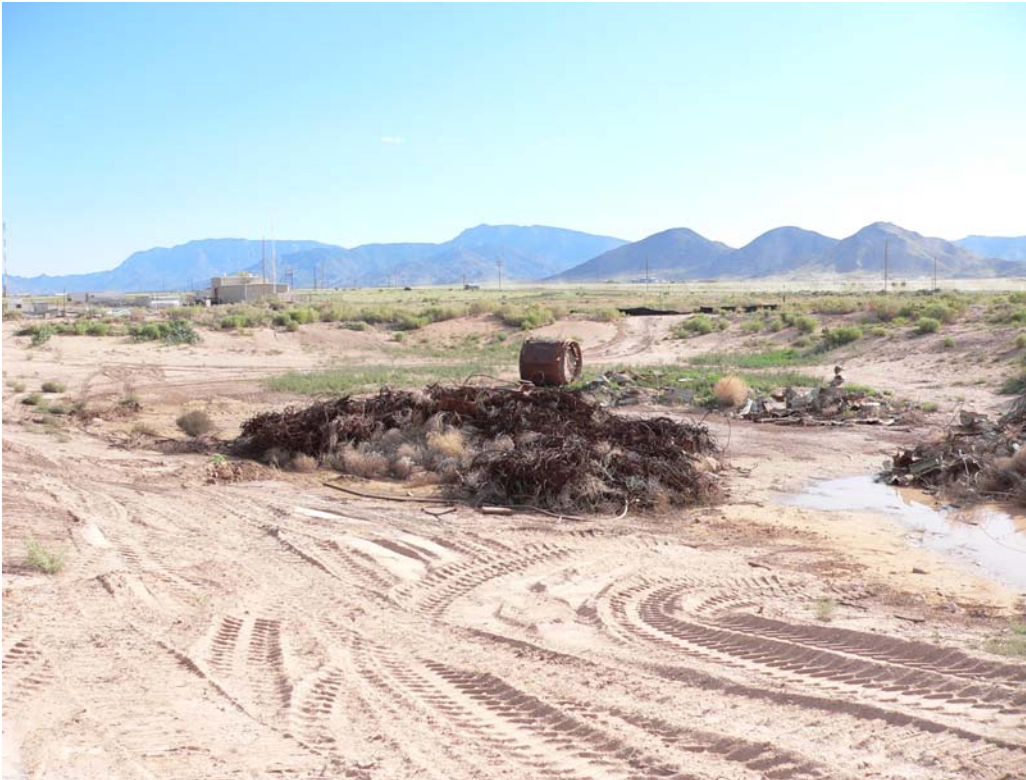
LTES Site 1 Metal Cable Piles Pre-Debris Removal
