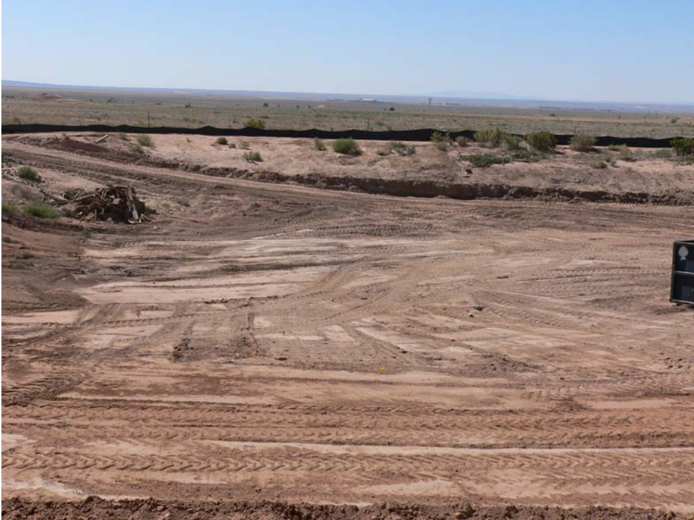
LTES Site 1 Post Debris Removal
