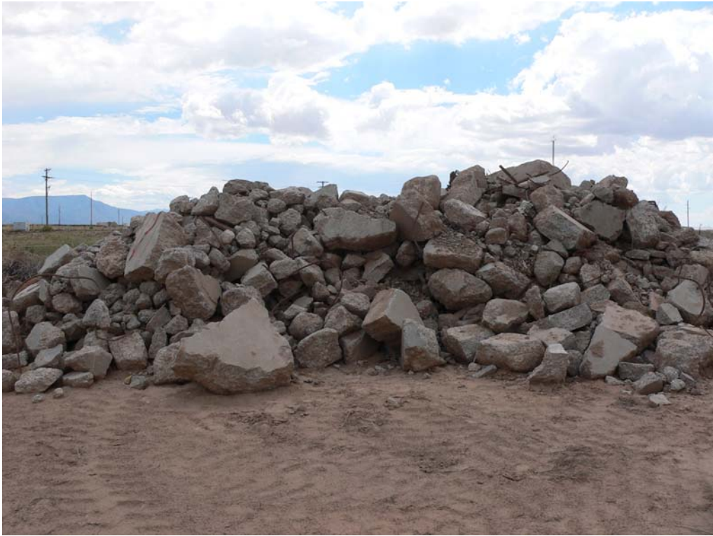
LTES Site 1 Concrete Staging Area
