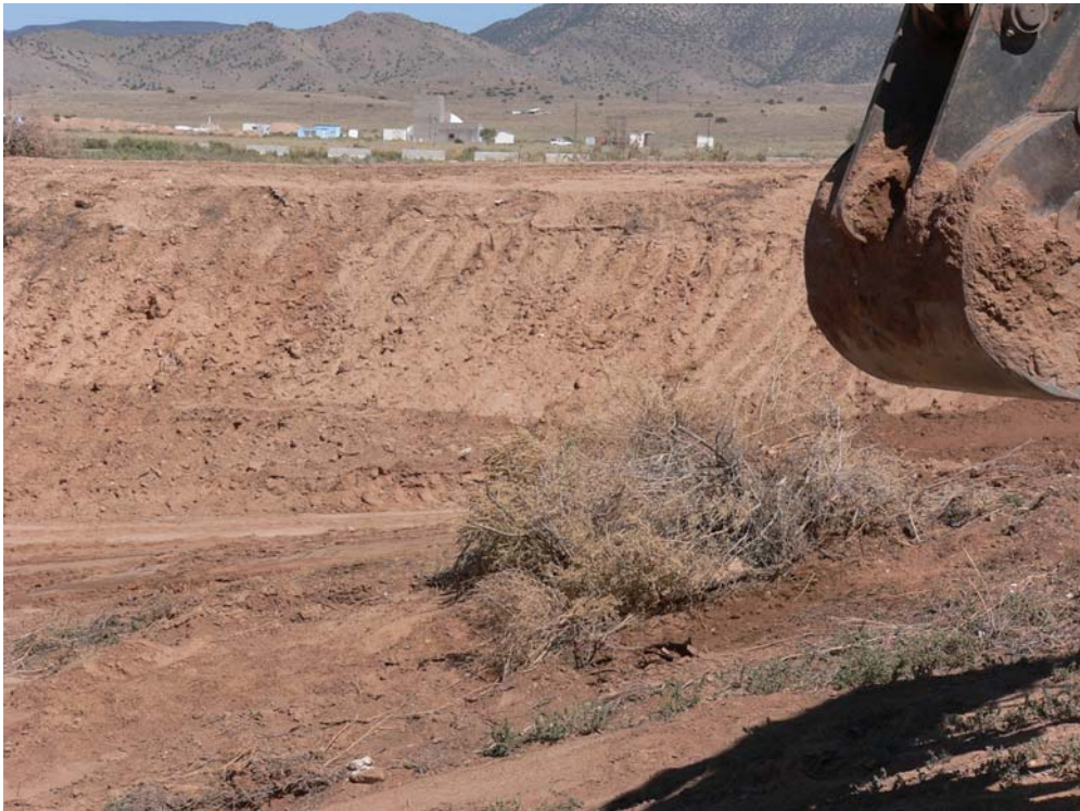
LTES Site 1 Post Debris Removal
