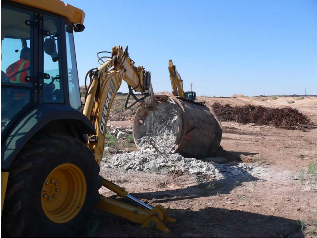
LTES Site 1 Steel Target Concrete Removal
