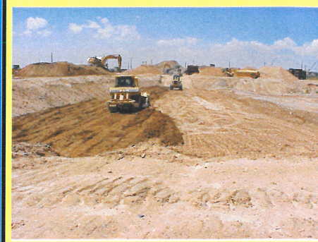
Backfilling VCM excavation..
