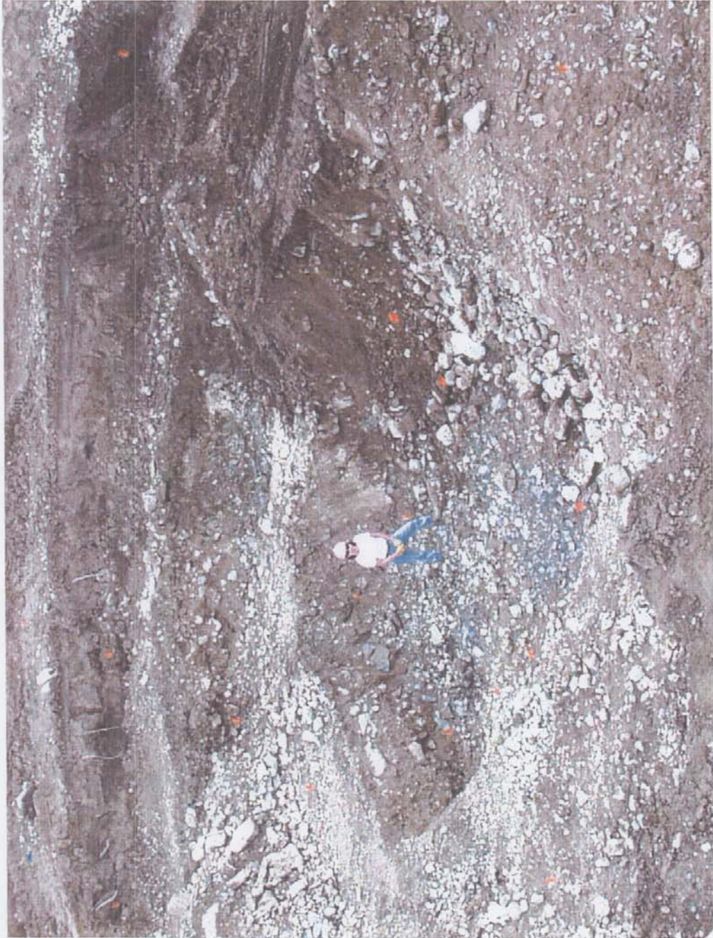
Figure 3.4.6-8 Finished Excavation Showing Top (in purple) of the Phyllite-Schist Bedrock
