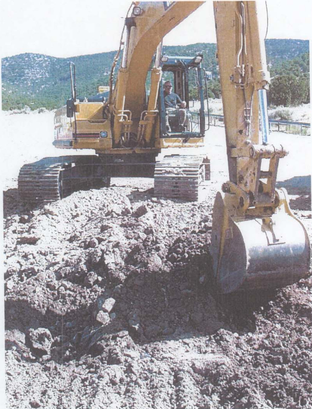
Figure 3.4.6-4 Excavator Removing First Lift of Clean Soil (view to the northeast)
