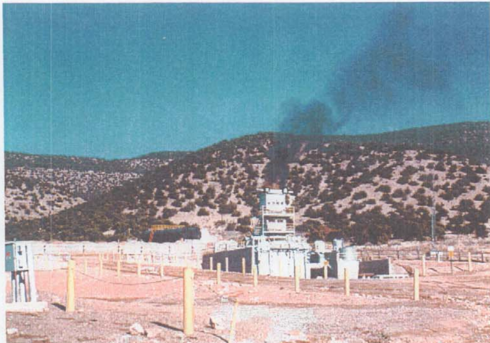
Figure 3A-10b Photograph of the SMERF conducting performance tests at SWMU 94 in December 1994. View is to the northeast.
