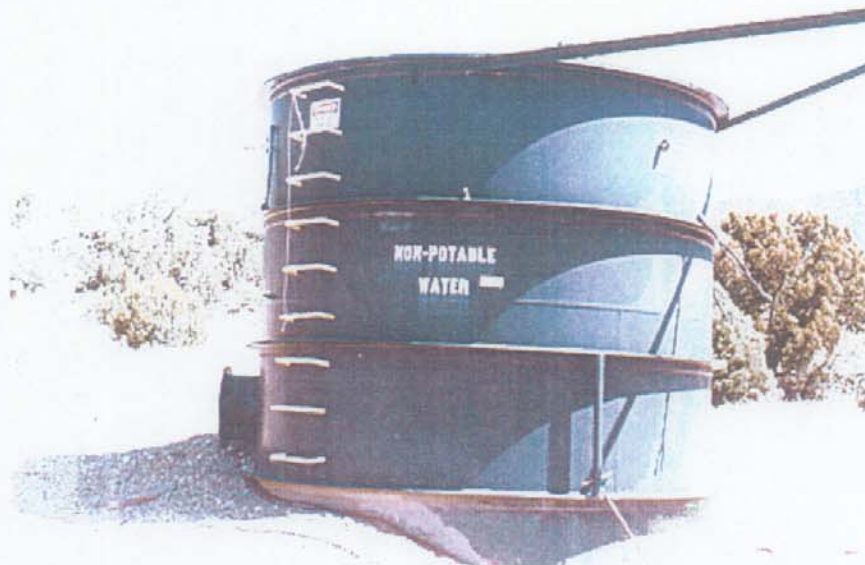
Figure 3A-11a Photograph of the above ground tank (SWMU 94A, Area 1) north of the LAARC Unit in April 1995. Additional above ground tanks storing fuel were located here when the LAARC was active. View is to the northeast.
