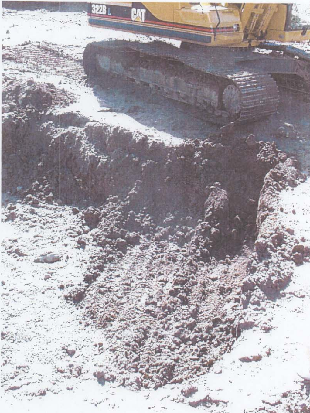
Figure 3.4.6-6 Excavating the Third Lift
