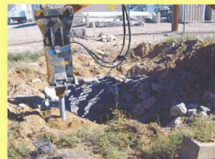
Seepage pit demolition and backfilling.
