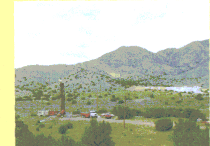
Drilling groundwater monitoring CYN-MW5 northwest of SWMU 49
