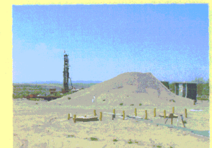
Drilling groundwater monitoring well CTF-MW2 northwest of SWMU 154 with the two HE seepage pits and an HE storage bunker in the foreground.
