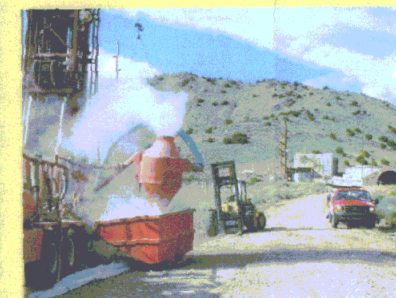
Drilling groundwater monitoring well CTF-MW1 southwest of SWMU 116. Drilling groundwater monitoring well CTF-MW2 northwest of SWMU 154 with the two HE seepage pits and an HE storage bunker in the foreground.
