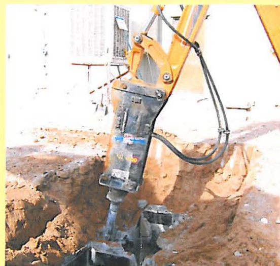
Septic system demolition and backfilling.
