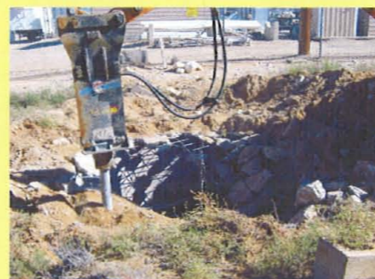
Seepage pit demolition and backfilling.
