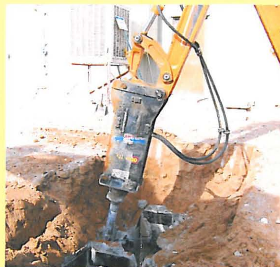
Septic system demolition and backfilling.
