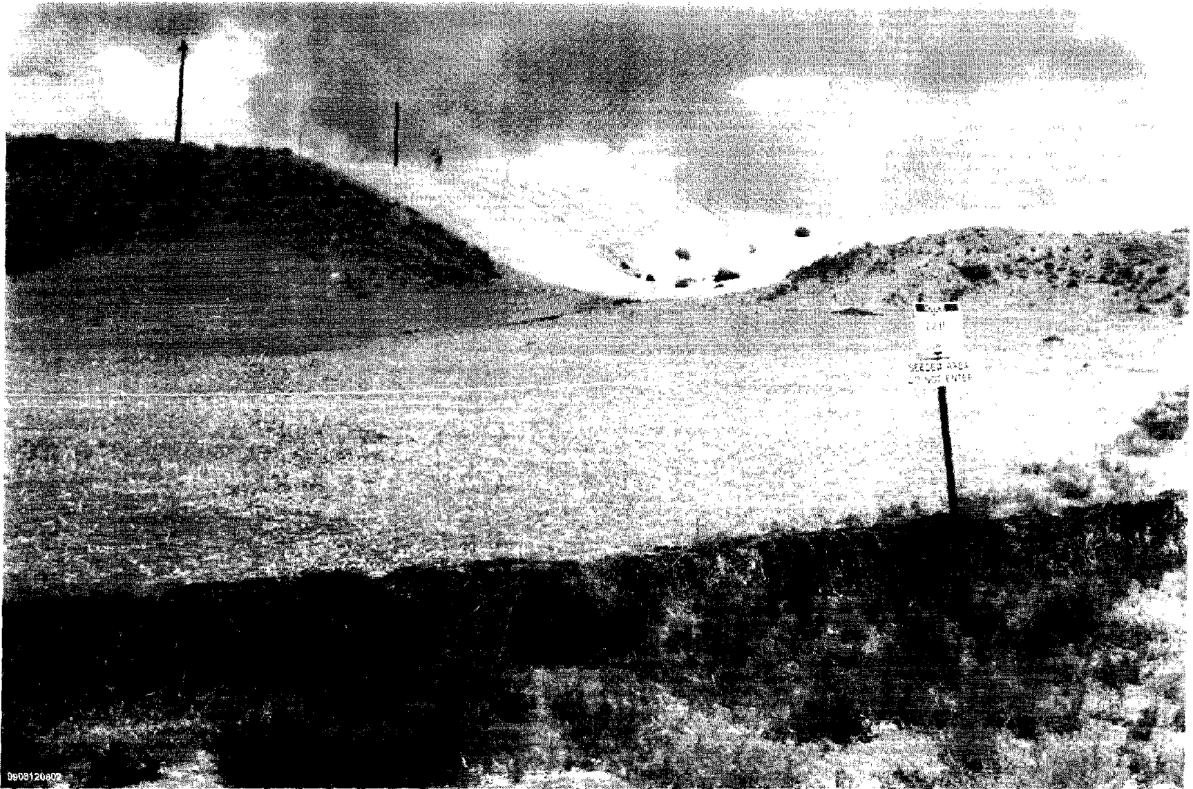
Figure 3.4.5-9 August 1999 photograph of SWMU 228A after final grading and revegetation work. View is to the northwest. Straw mulch is visible across the center of the site. Erosion control mats are visible in the gully.
