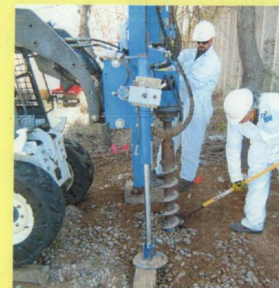
Auger drilling through the gravel aggregate to collect additional soil samples for VOC analysis at the AOC 1117 Drywell.
