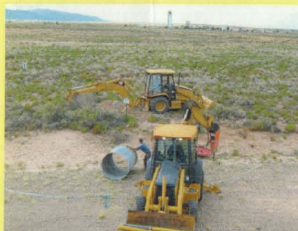
Backfilling the seepage pit excavation at AOC 1095. The section of metal culvert that was removed from the seepage pit is next to the worker in the foreground. The Solar Tower is in the background.
