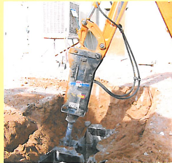
Septic system demolition and backfilling.
