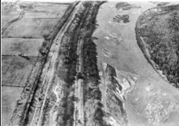
Fig. 9(a): Location of the jetty installation. Photo: Dec. 12, 1952.
