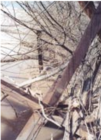
Fig. 14: The MRGCD wants riverbank jacks to stay in place for levee protection
