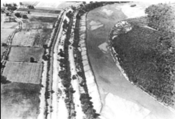
Fig. 9(b): Jetty field installed. Photo: Aug. 12, 1953.
