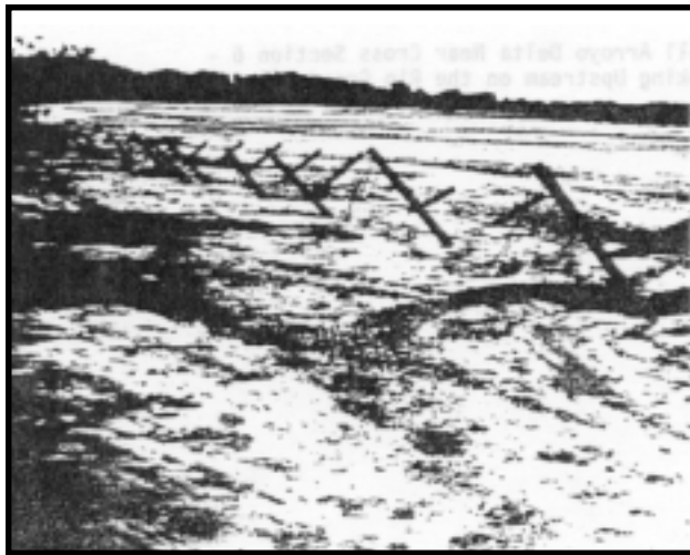
Figures 23-24: Before and After: At left is a jetty jack installation at Santa Ana, photo 1974 (Lagasse 1980). Below is the result of bank restoration using bio-engineering methods and native willow planting.
