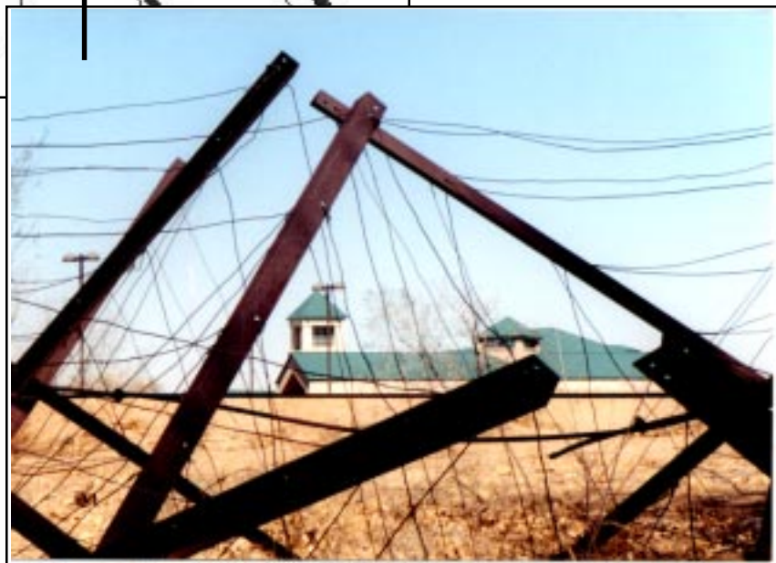
Fig. 20: Jetty jacks dominate the bosque near the levees. Many of these will stay in place in the Rio Grande Valley State Park. Note the BioPark in the background. The endangered silvery minnow is being bred in captivity in the facility's aquarium.
