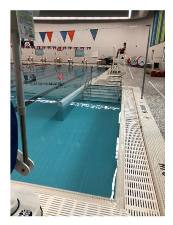
As for the design of the pools, he explained differences in their gutter design, such as keeping the gutter in the family pool flush with the deck to prevent tripping, because the primary users of the pool were seniors and children. He also explained the design concepts for the pool edges:
