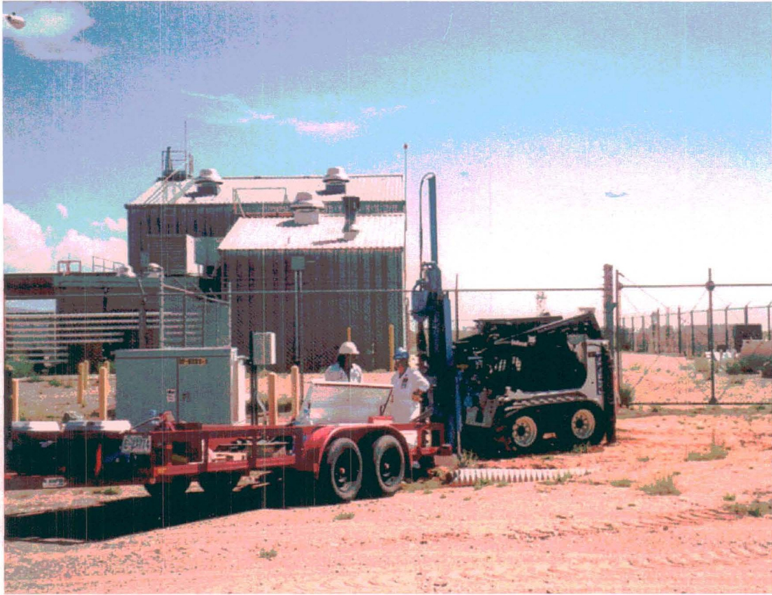
Figure 3.4-1 Collecting soil samples in the DSS Site 1007, Former Building 6730 Septic System Drainfield. View to the south. August 16, 1999
