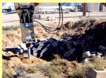
Seepage pit demolition and backfilling.
