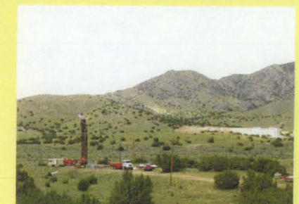
Drilling groundwater monitoring CYN-MW5 northwest of SWMU 49
