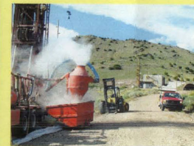
Drilling groundwater monitoring well CTF-MW1 southwest of SWMU 116.
