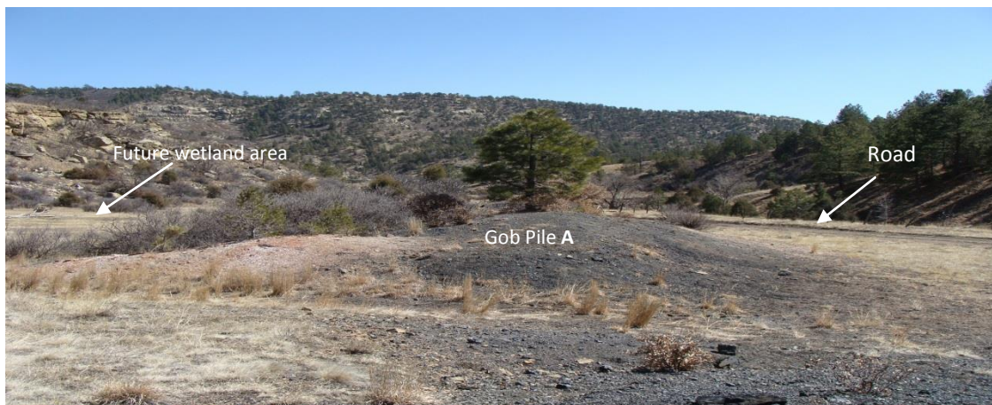
Figure 5: Standing at downstream edge of second pond looking east (2009 EA)
