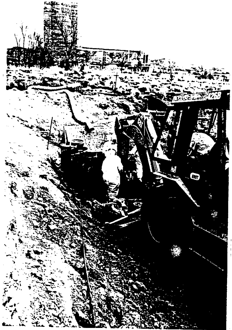
Below: Building 9980 septic tank septage removal and tank cleaning operation. October 24, 1995 View looking east.
