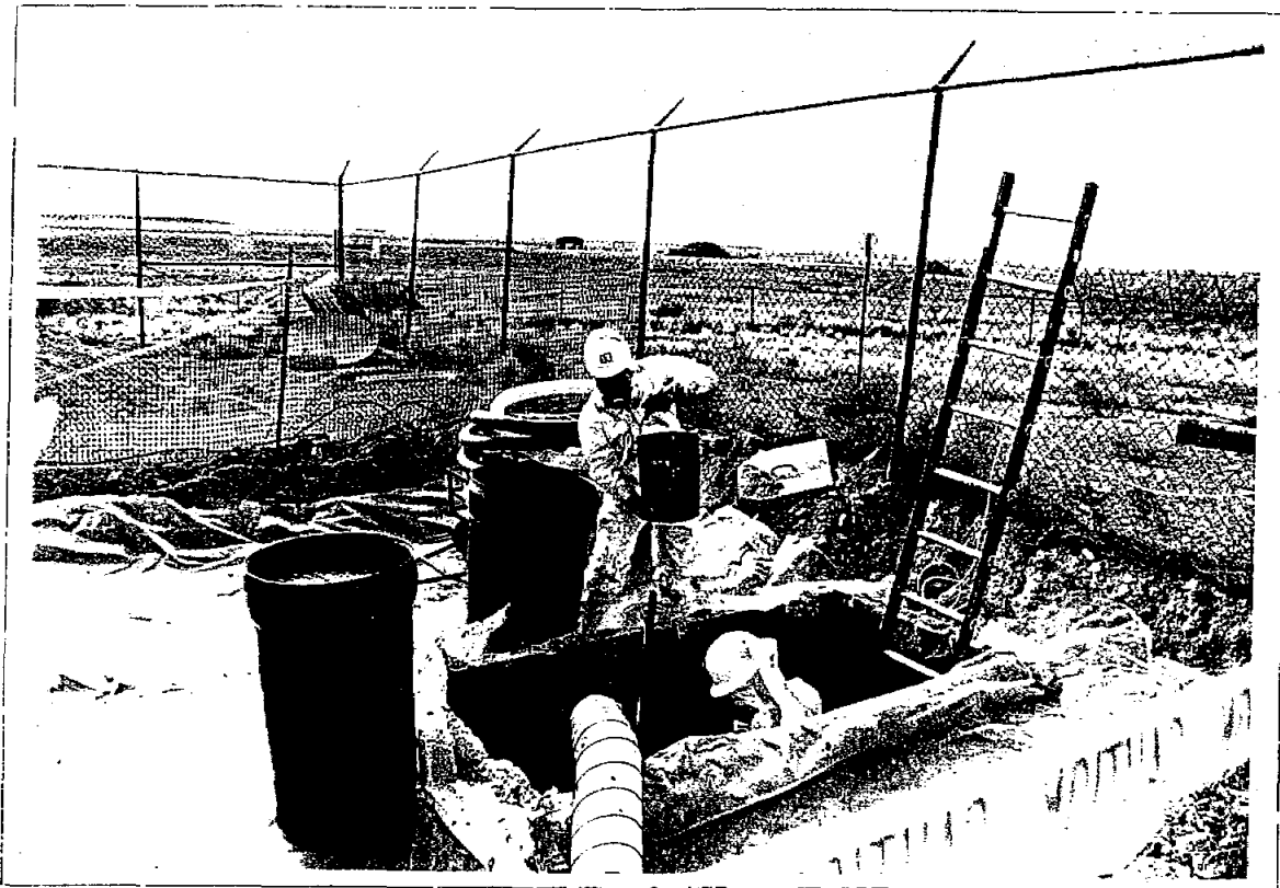
Building 9965 septic tank septage removal and cleaning operation, December 12, 1995. View looking southwest.
