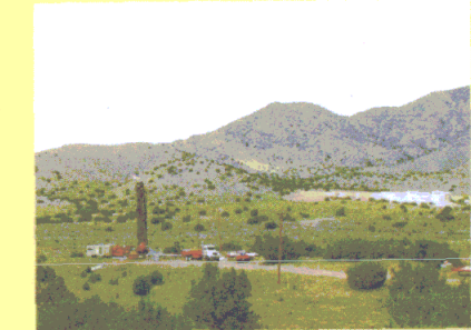
Drilling groundwater monitoring CYN-MW5 northwest of SWMU 49
