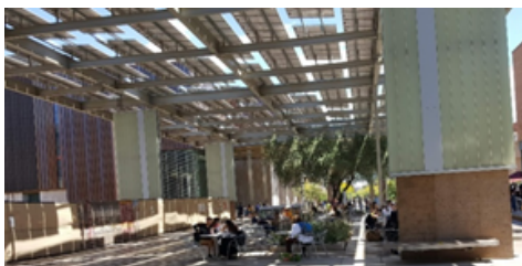
Fig. 6. Solar panels over walkways at ASU Tempe Campus, AZ, USA.
