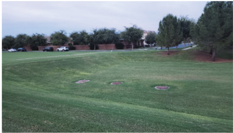
Figure 2. A retention pond in a residential development,
