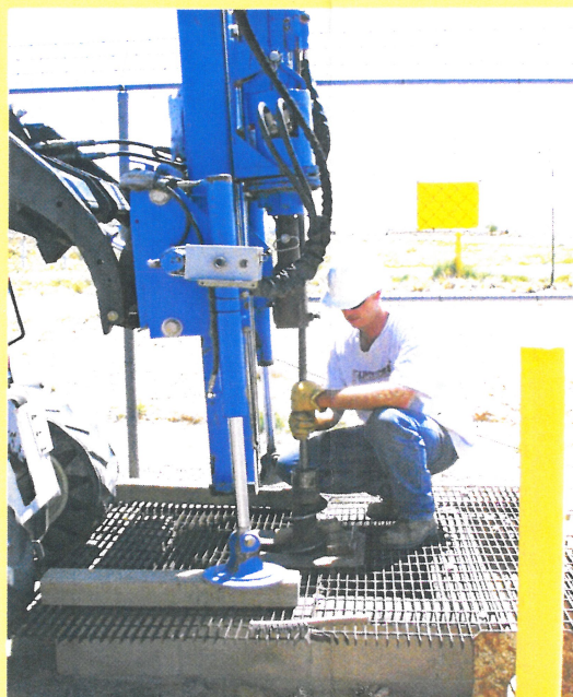
Platform and Geoprobe sampling equipment used to collect soil samples from beneath the center of the seepage pit.
