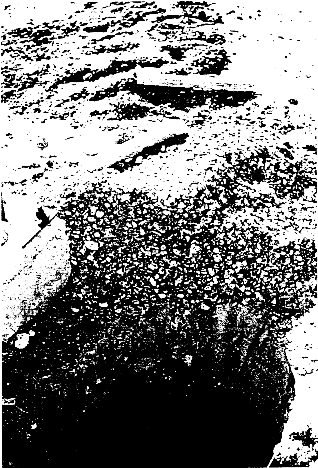
Figure 1-3 Photograph of Excavation of SWMU 111 Gravel Pit, 1988
