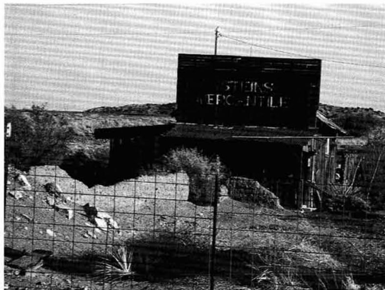
Mercantile store and adobe ruins at Steins Ghost Town (June 6, 2011, photograph by Carleen Lazzell)
