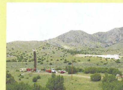
Drilling groundwater monitoring CYN-MW5 northwest of SWMU 49
