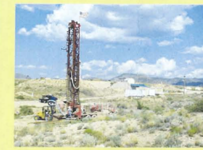
Drilling groundwater monitoring well CTF-MW3 west of SWMU 149
