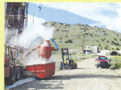
Drilling groundwater monitoring well CTF-MW1 southwest of SWMU 116. Drilling groundwater monitoring well CTF-MW2 northwest of SWMU 154 with the two HE seepage pits and an HE storage bunker in the foreground.
