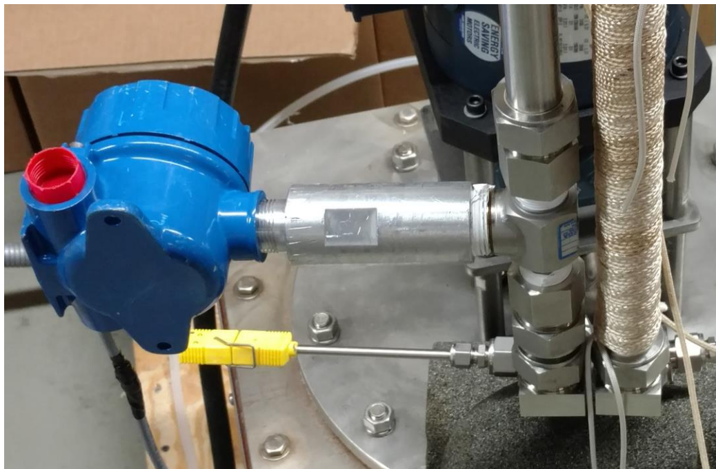
Figure 3-7 Omega FTB-1400 flow meter with signal conditioner
