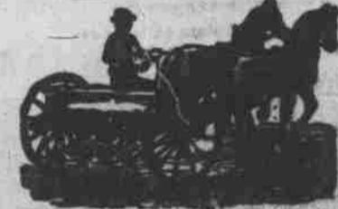
Our Buckeye Drills can be adapted to all kinds of soil, as to weight, capacity, number of hoes, and size of wheel, so as to make them the most efficient and economical pieces of machinery ever put into the market.
