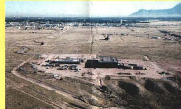
Low-altitude oblique aerial photograph showing construction of TA-IV in 1978. Storm water ditch is visible at lower left corner of photograph. The three SWMU 46 outfall ditches are faintly visible and are located between the storm-water ditch and Buildings 980 and 981. View to North, 1978.
