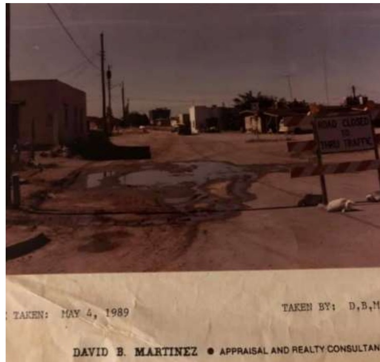
FIGURE 13 CAMPO STREET, “MY MOM’S HOUSE WAS DEMOLISHED WEEKS AFTER THIS PICTURE WAS TAKEN. THE POLICE DEPARTMENT IS NOW SITTING WHERE WE ONCE LIVED.” PHOTO AND QUOTE BY ANNA SALAZAR
