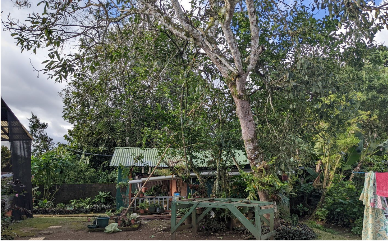
Figure 26: A "rancho" structure which was part of my family's first dwelling in the area.
