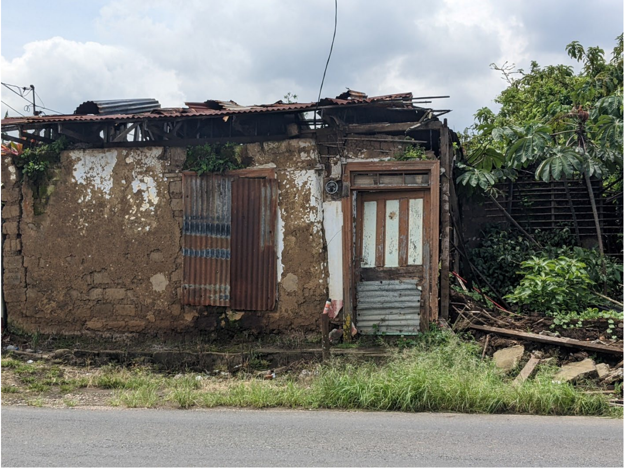
Figure 21: A traditional adobe structure in San Ramon, Heredia.
