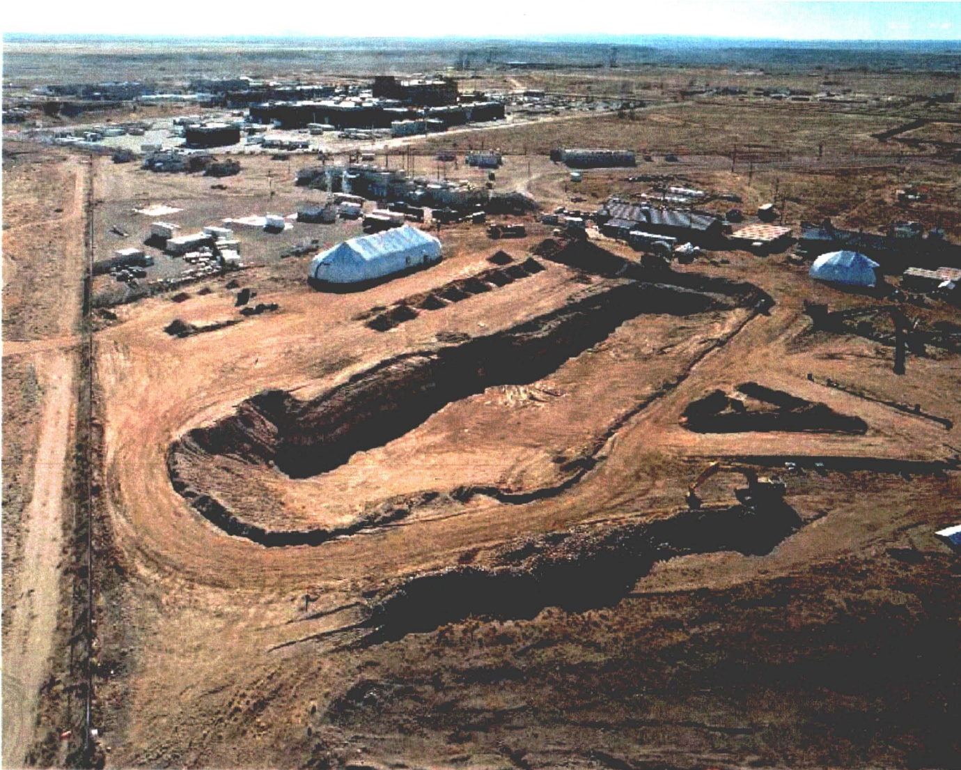
Figure 5.6.2-1 SWMU 2 During the VCM Excavation, View to the Southwest
