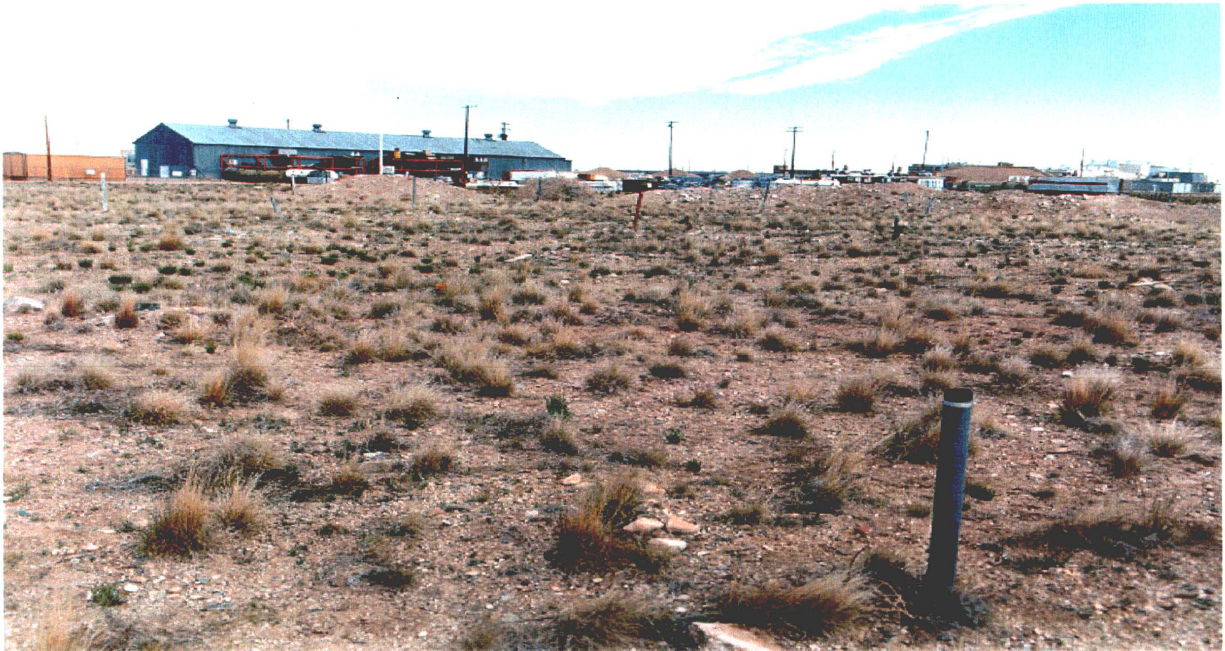
Figure 5.2.2-2 View to west across SWMU 2 prior to the VCM showing steel pipe steel markers for disposal cell and trench locations
