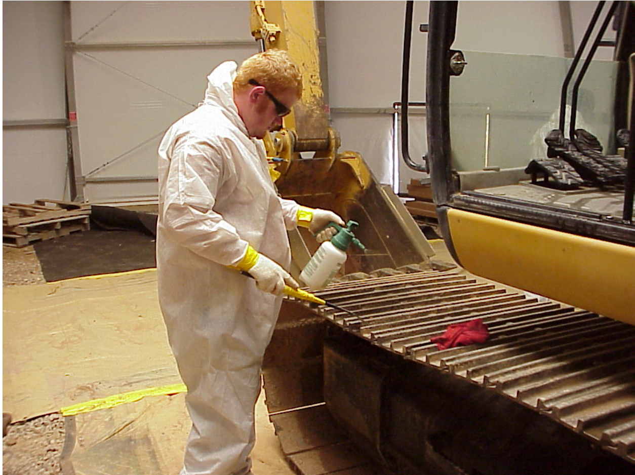
Figure C-2 Personnel Performing Decontamination of the Excavator, August 7, 2003
