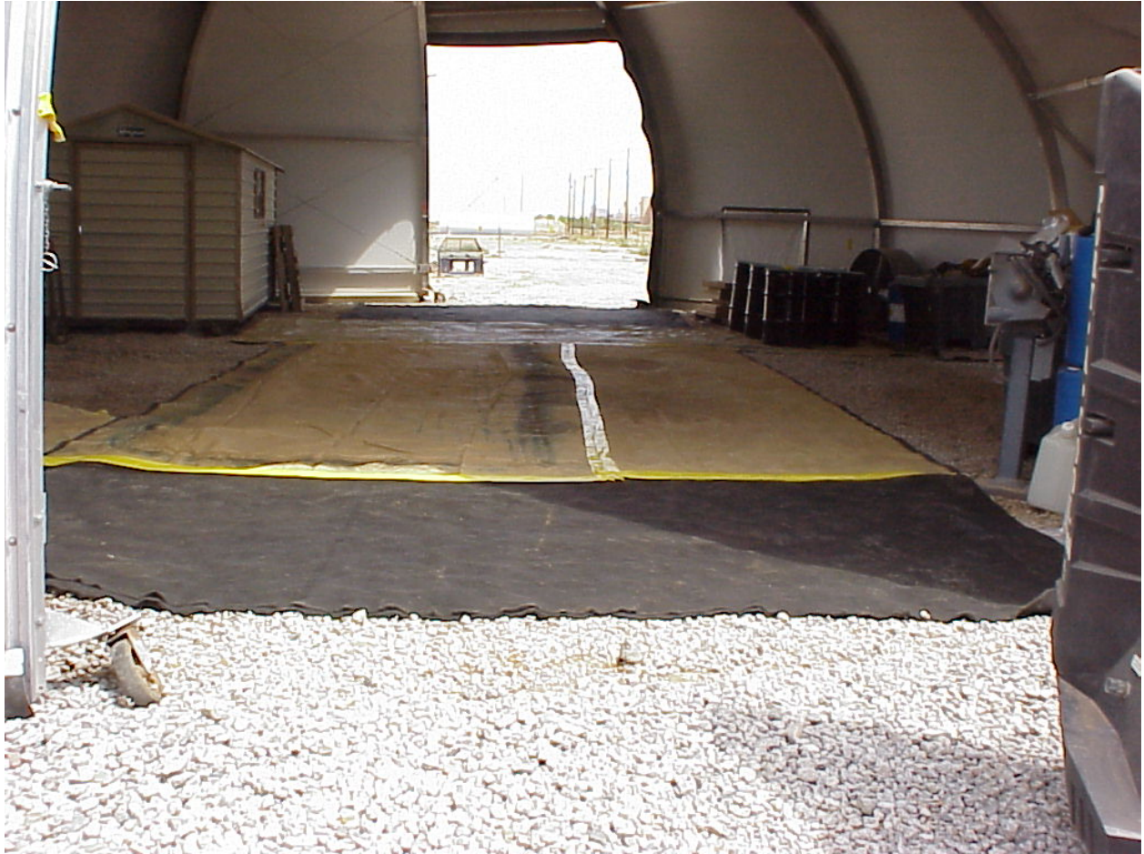
Figure C-1 Classified Waste Landfill Decontamination Pad, August 6, 2003
