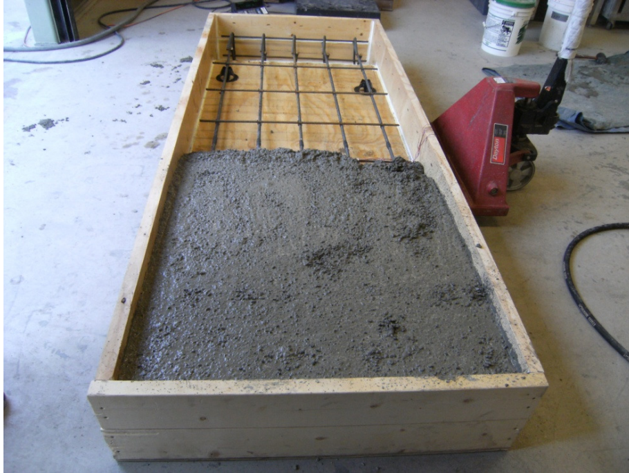
Figure 3.13: Casting the control slab
