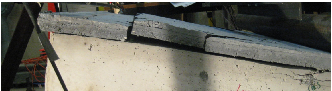
Figure 5.18: Horizontal shear failure of the UHPC outside of the shear-friction reinforcement (profile)
