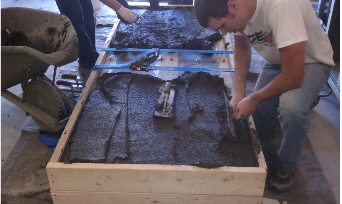
Figure 3.26: Casting the first UHPC batch
