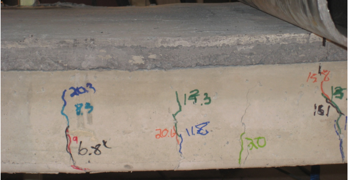
Figure 5.14: Strengthened slab prior to UHPC debonding
