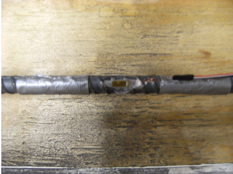
Figure 3.16: Strain gauge on a reinforcement bar
