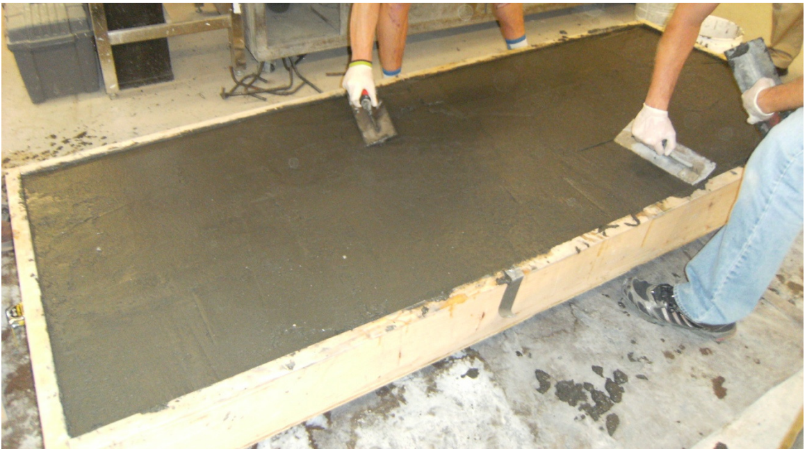
Figure 3.27: Finishing the second UHPC batch
