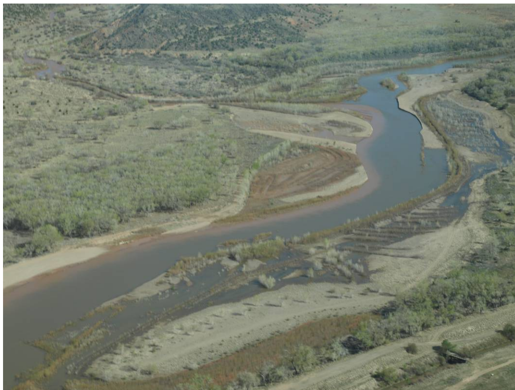
Photo 8: Bank erosion upstream of the GRF wingwall (2011, AuBuchon)
