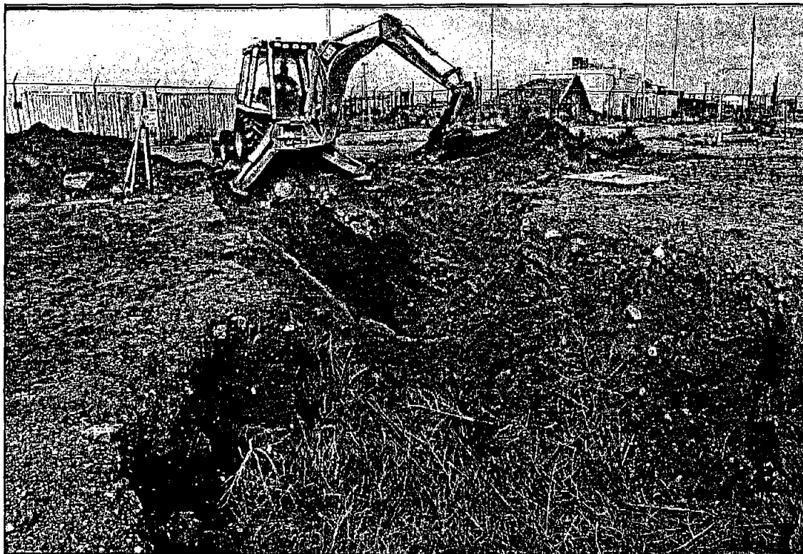
Figure 8 Backhoe digging exploratory excavation at western end of SWMU 229 outfall ditch. (TA-II visible in right background, TA-IV visible in left background. View to northwest, February 2001.)
