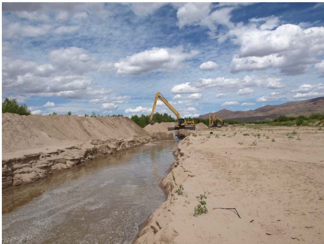
Photo 4: Excavation of pilot channel through Temporary Channel sediment plug. Taken approximately ½ mile downstream of Red Rock Staging Area, looking upstream (September 2009, Rolland)
