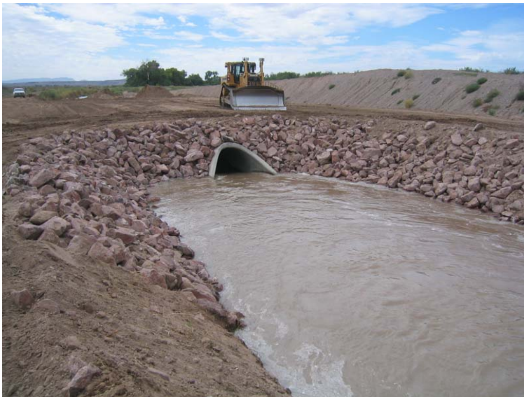
Photo 7: Elmendorf Drain culvert replacement, showing the new 84-inch diameter concrete pipe, looking downstream (October 2009, Everetts)
