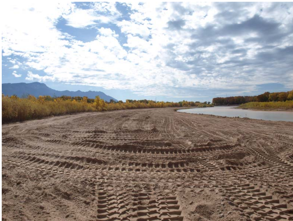
Photo 14: Looking downstream at location of sediment spoil pile on the Pueblo of Santa Ana after sediment has been removed. Flow in the Rio Grande is approximately 500 cfs (October 2009, AuBuchon)
