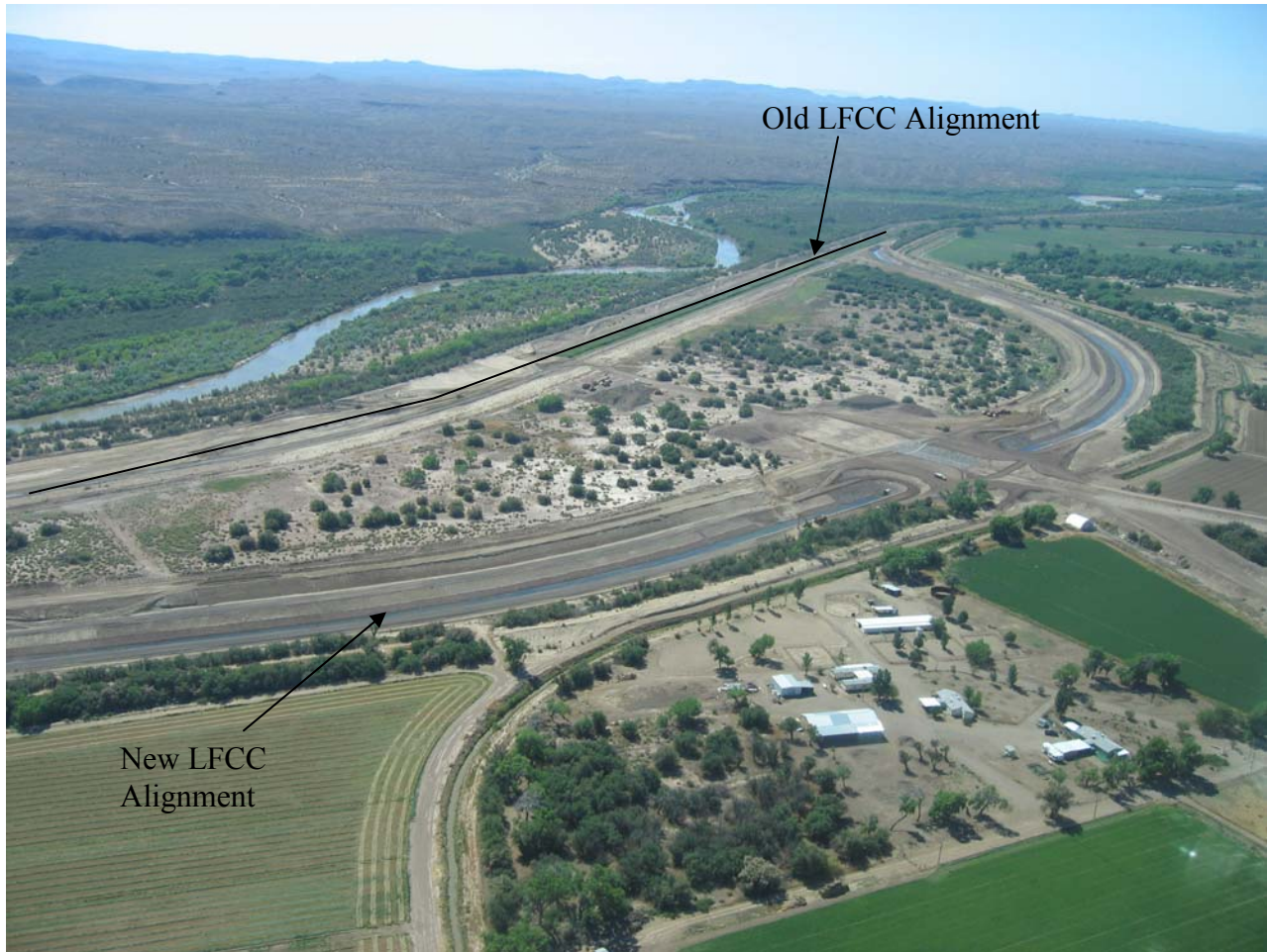
Photo 8: Looking downstream at the new LFCC in the area of River Mile 113/114 Priority Site (May 2006)
