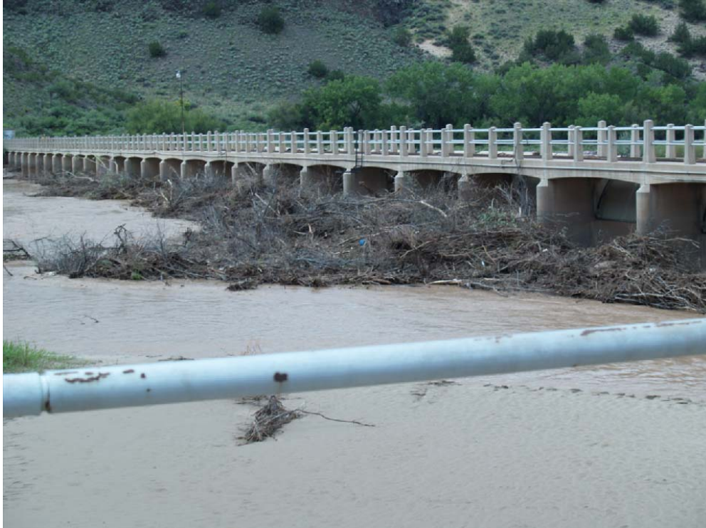
Photo 14: Debris removal at San Acacia Diversion Dam
