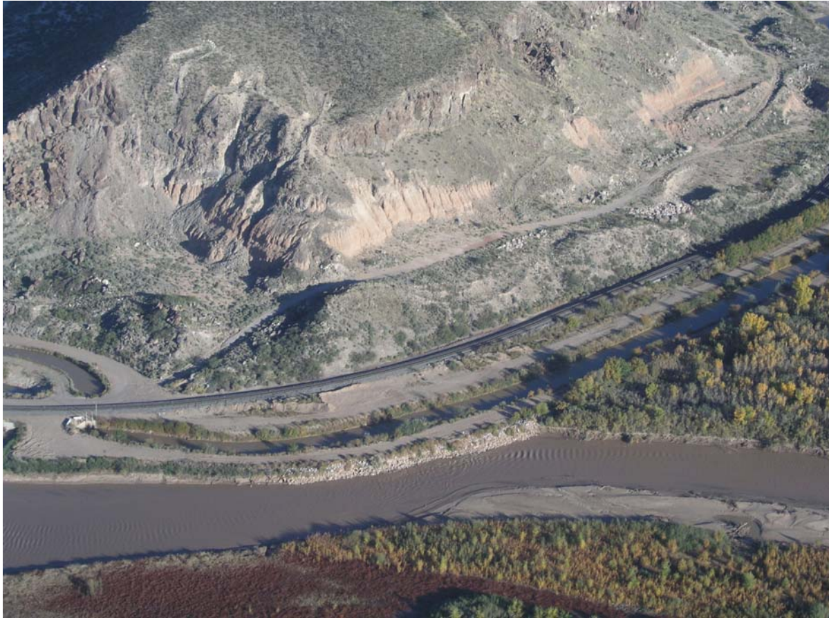
Photo 7: Drain Unit 7 priority site (October 2006)
