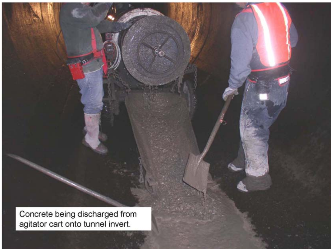
Photo 1: Concrete being discharged from agitator cart onto tunnel invert (2006)
