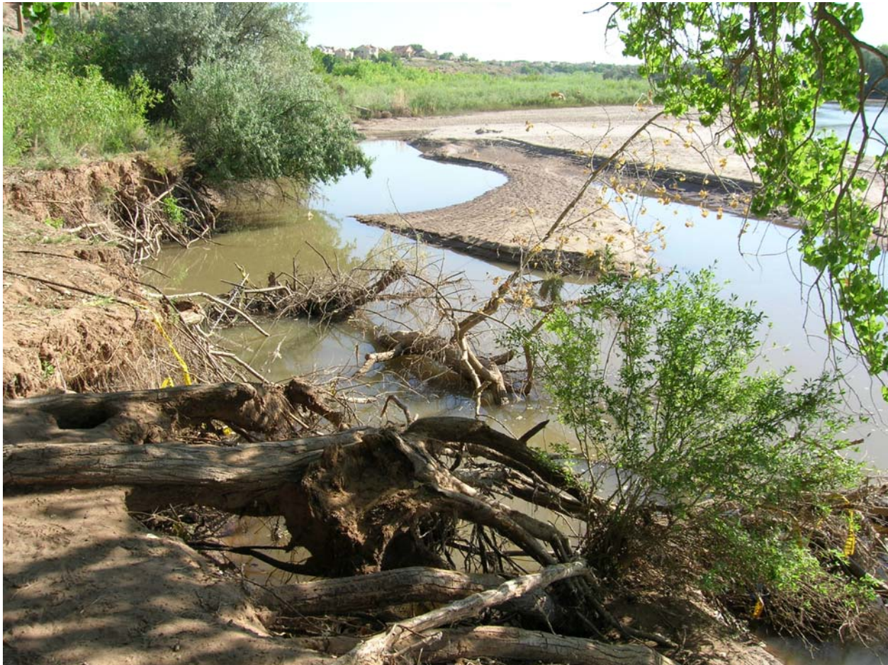
Photo 6: Bank erosion at the Corrales Siphon priority site (July 2005)
