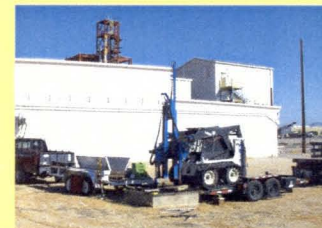
Collecting soil samples with the Geoprobe.
