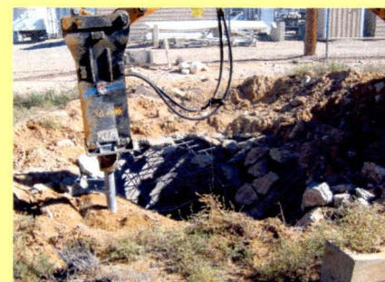
Seepage pit demolition and backfilling.
